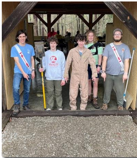
Arrowmen re-pave path at Camp Coker
